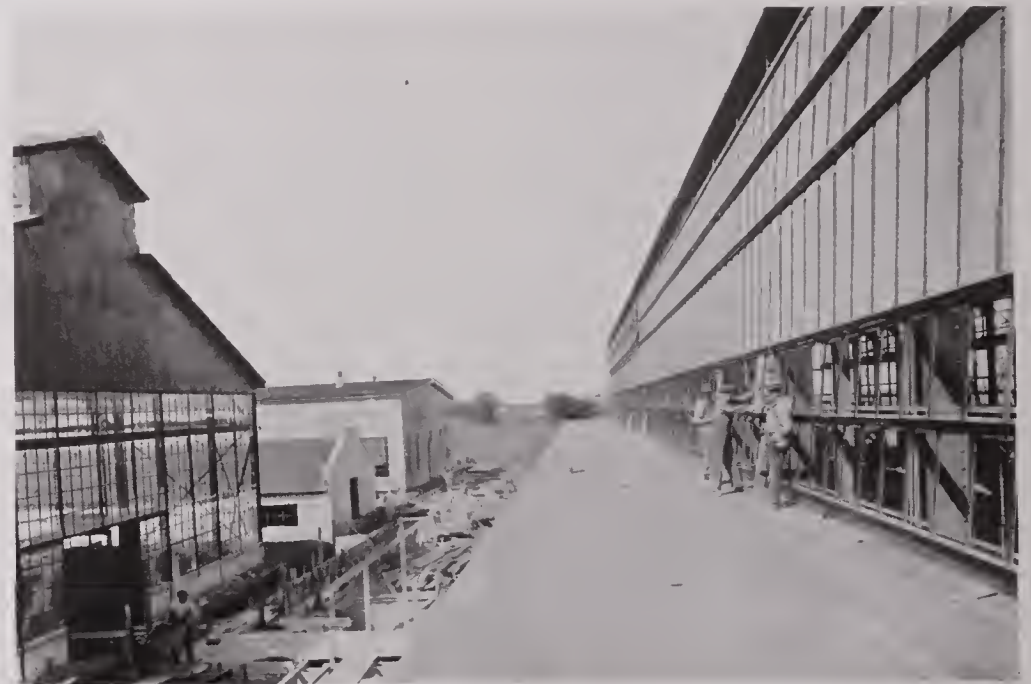
FROM HAMMER SHOP ROOF
